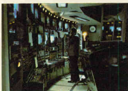
Master control engineer adjusts test signals in preparation for network test.
