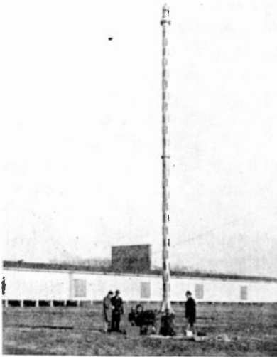
Fig. 2—Antenna installed in the normal vertical position in a rotating socket for measuring horizontal patterns.
