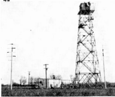
Fig. 3—The receiving equipment site at Brandywine, near Wilmington, Delaware.
