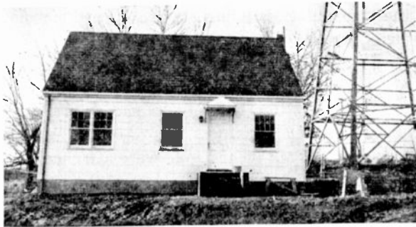
Fig. 3—Transmitter Building (front view).
