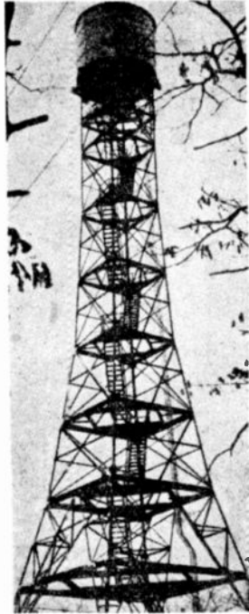
Fig. 3—Hauppauge tower and penthouse.
