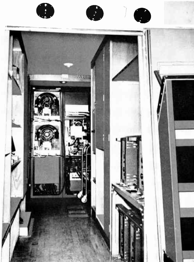
FIG. 28. General storage area of mobile unit as seen through rear door.
