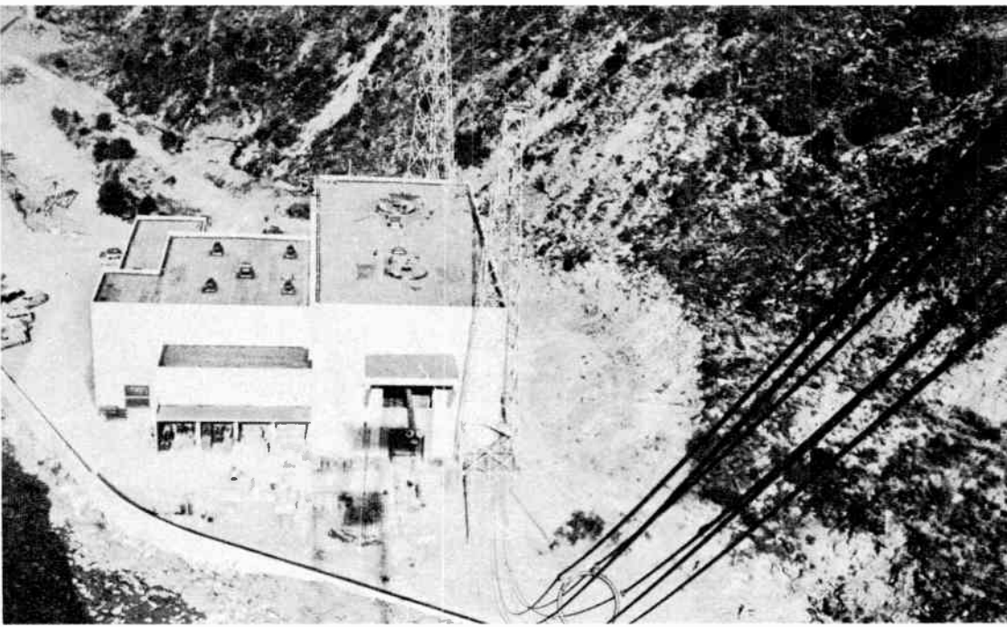
Navy's Jim Creek station, as seen from one of its 200-foot towers. At right is a six-wire "cage" antenna lead dropping to the building that houses transmitter. Antenna system uses 30 miles of wire.
