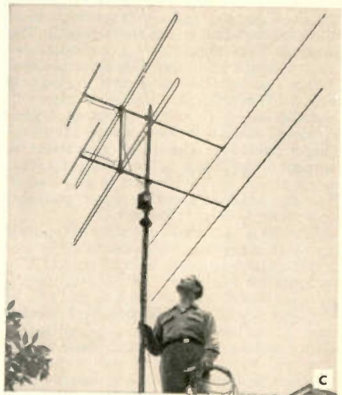
Two-bay stacked array with motor-driven rotating device to turn the TV antenna in any direction
