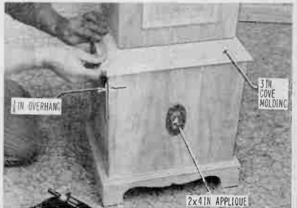
Cove molding and applique are best applied with hot glue: it sets in just 60 seconds.
