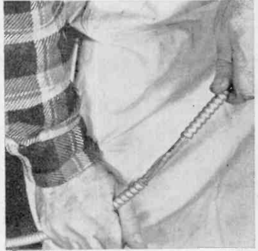
Break the sheathing by twisting and bending where it was notched with hacksaw. Pull cord to split paper.
