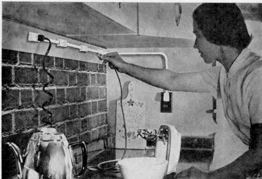
Plenty of convenience outlets are needed to provide current for the many appliances used to prepare meals.
