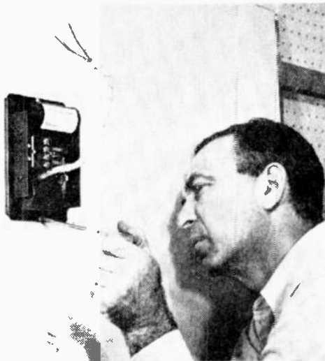
FIG. 1: Converting from a bell or buzzer to chimes requires a larger transformer for higher voltage.
