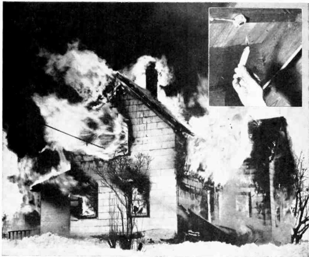
Early warning might have prevented this. Alarm box can be mounted out of way in bedroom near regular receptacle. Heat sensitive detector, inset, set for 140°, can be positioned over likely trouble spots.
