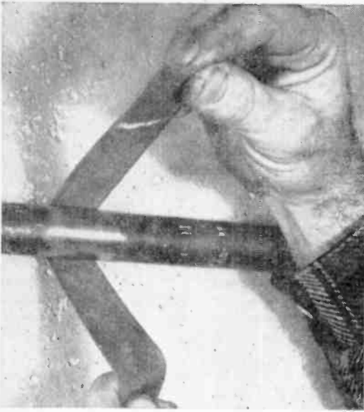
Use emery cloth to sand the pipe down to bare metal before attaching clamp that will ground appliances.
