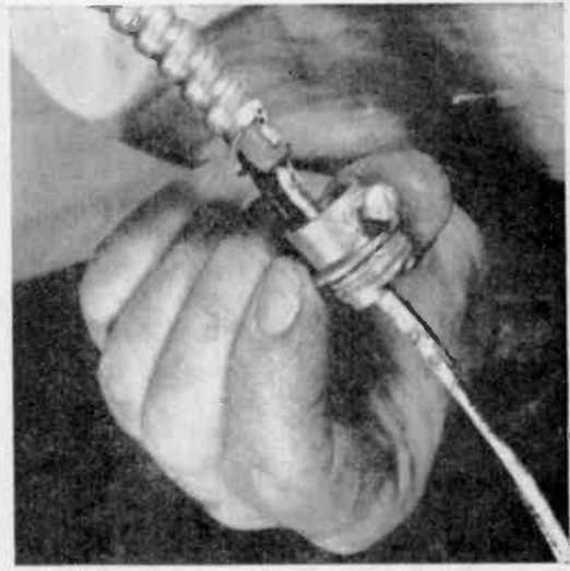
Connector slipped over cable armor and locked by tightening set screw, will hold the wire to junction box.
