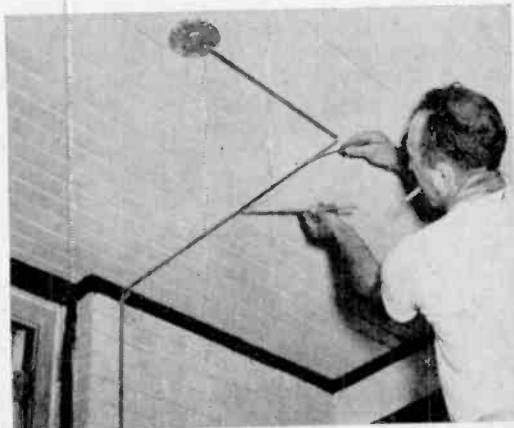
Lamp holder has a special plate to which surface fixture is attached. Paint channel to blend with ceiling.
