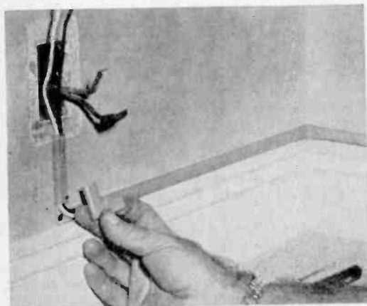
Plate will cover the opening once wires are spliced. Corner cap snaps over the metal channel for a neat fit.
