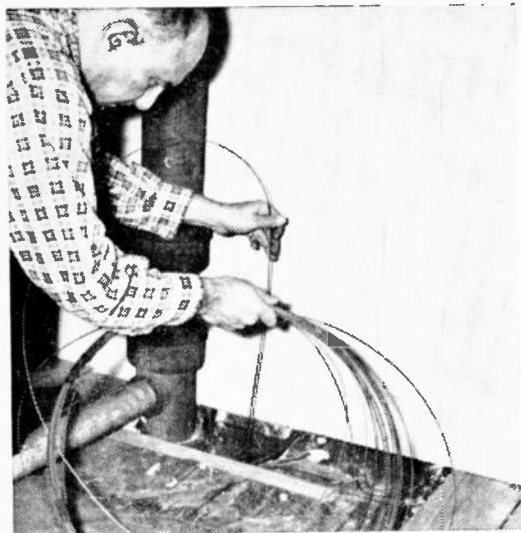
First place to consider snaking the fish tape is along-side the soil stack where an opening usually exists.
