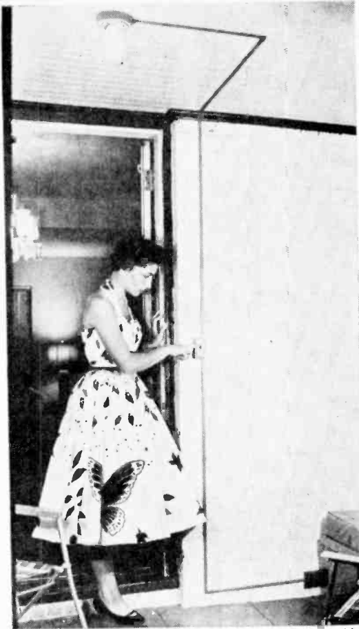
Extra outlets, switches, lights, etc. can be quickly installed with channel ducts that have snap-on covers.
