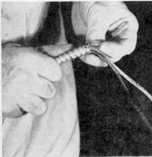
Protect wire insulation from jagged end of the cable by pushing a round fiber washer into the open end.
