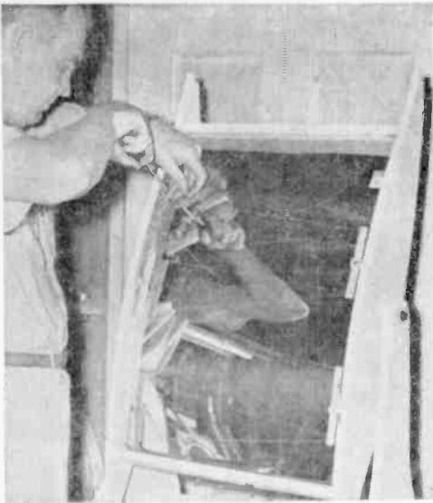
FIG. 5. Attaching heating element to supports. Stretch to 80 in. before installing.
