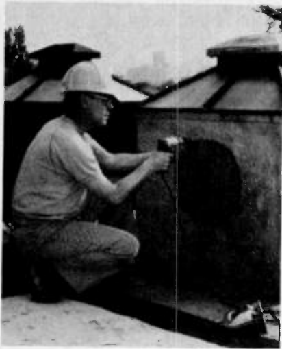
Position the cardboard template to mark the size and position of the desired cutout. Use a saber saw, or drill holes on the line.
