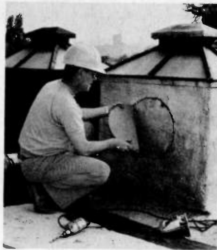
The cardboard template is pulled free and we see the drilled holes. A hammer and chisel finally freed the outlined disc.
