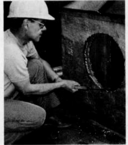
When we came to an obstructing stud, we used a keyhole saw to remove it, but you could use just about any small saw.
