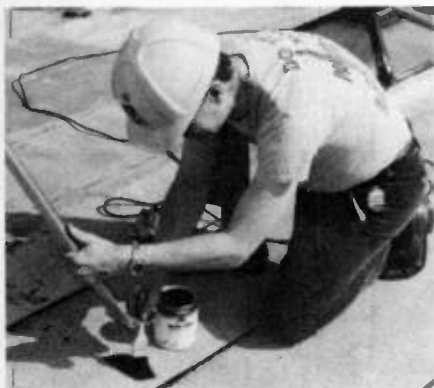
Use roof patch compound to prevent rain-water leakage through the pilot holes.
