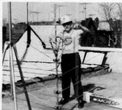
Unpack the antenna on the roof and unfold the elements only when you are ready.
