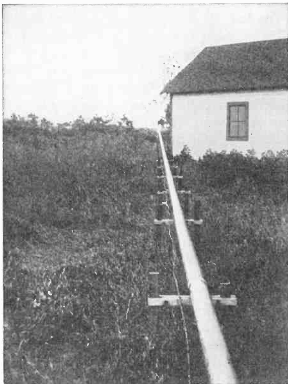
Fig. 9.3 A section of the first experimental waveguide transmission line built at the Netcong, N.J. receiving site in August, 1933.
