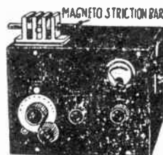
Magnetostriiction Oscillator
