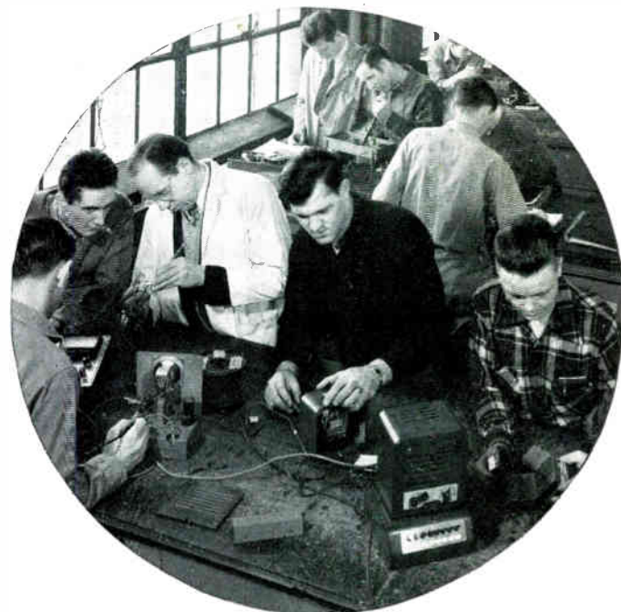
In the picture above, you see a Coyne instructor explaining and demonstrating on an Inter-Communication system. This is a branch of Electronics that is becoming more and more popular. Thousands of them are already in use in business concerns and offices of various different kinds and the demand for this equipment is constantly increasing.
