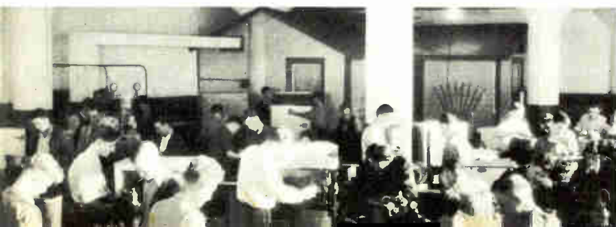
This picture, taken in our Electric Refrigeration Department, shows Coyne students carrying out the series of operations involved in the overhaul on a compressor and motor combination unit.
