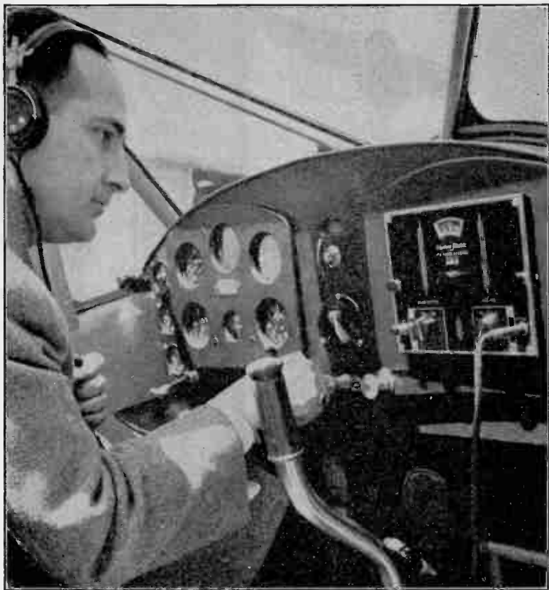
FIG. 2—Illustrating aircraft radio receiver. The pilot receives code and messages through head phones which are interconnected to receiver as shown. (Courtesy Western Electric Co.)
