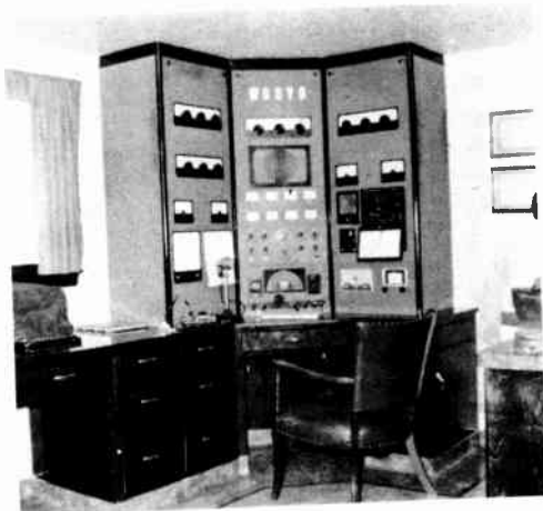
This neat "built-in" installation features separate finals and exciters for each band, along with room for receiver, frequency meter, oscilloscope, Q multiplier and v.h.f. converter. All units are mounted on the three large panels; the panels are hinged at the bottom so that they can be lowered for service work on the individual units. A common power supply is used, and band-changing consists of turning on the filaments in the desired r.f. section. (W9OVO, Sturgeon Bay, Wisc.)
