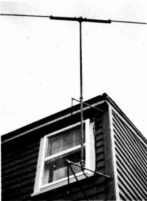
Fig. 14-61—Over-all view of the antenna and mounting. The feedline comes out of the bottom of the mast and through the wall into the shack.
