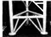
Connecting point of C-20 and C-25 towers.
