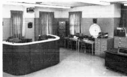
An overview of the W1AW station. The main operating console on the left houses the control equipment for simultaneous code practice/bulletin transmissions on eight bands. Two visitor operating positions are on the right.
