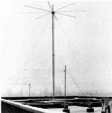
Fig. 39 — The completed discone antenna, installed on the roof of a three-story building.
