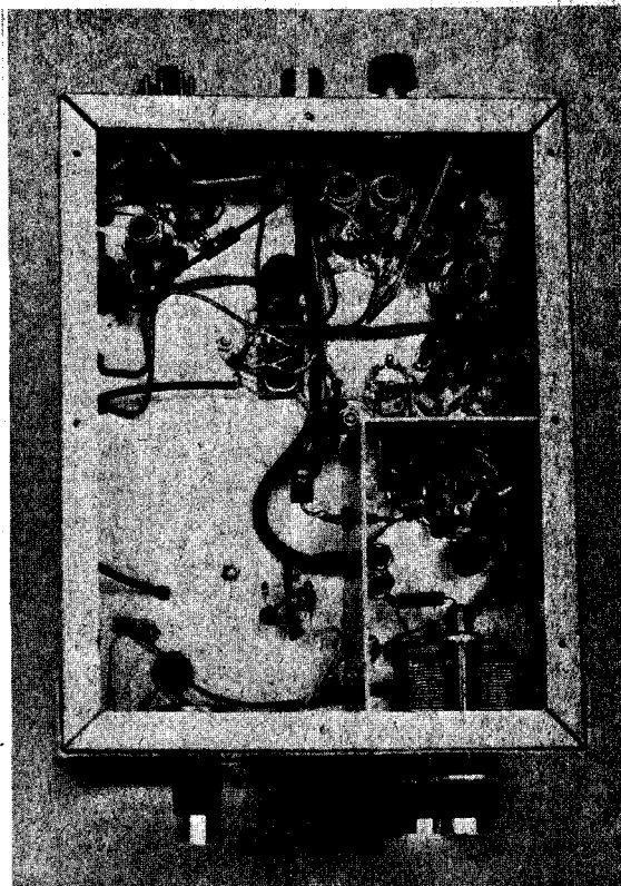
Fig. 7-6 — Bottom of the transverter, with the 6146 socket inside the shield compartment at the right. Three sets of inductively-coupled circuits are visible in the upper-right corner. The first two, near the top of the picture, are on 22 MHz. Next to the right and down, are the mixer plate and first-amplifier grid circuits. The self-supporting 6GK6 plate and 6146 grid coils are just outside the amplifier shield compartment. The large variable capacitor is the loading control.
