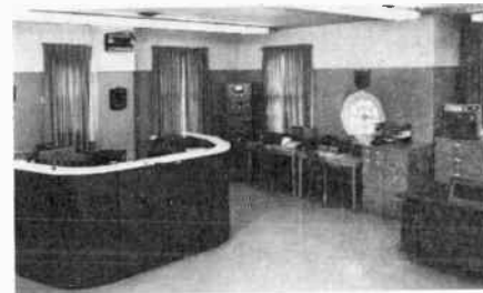
An overview of the W1AW station. The main operating console on the left houses the control equipment for simultaneous code practice/bulletin transmissions on eight bands. Two visitor operating positions are on the right.
