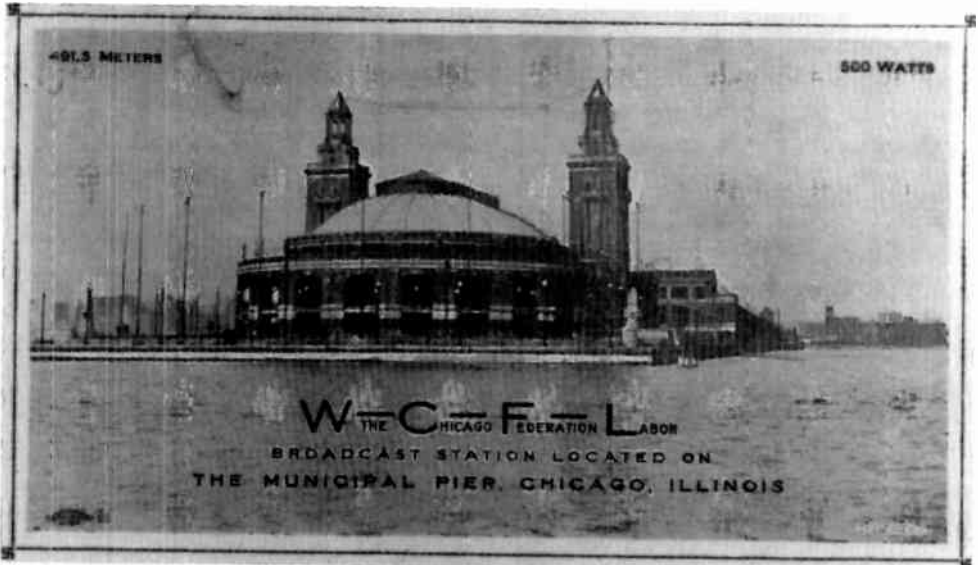
Workers from various Chicago trade unions erected a transmitter and installed the equipment for a WCFL studio in the north tower at the east end of Navy Pier in 1926. WCFL began regular broadcasts on July 27, 1926. This illustration is from the CFL letterhead, circa 1926. (Courtesy of the Chicago Historical Society)
