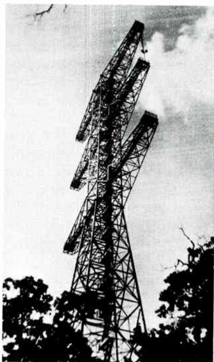
Completed tower: W 2 XMN—1938. Columbiana
