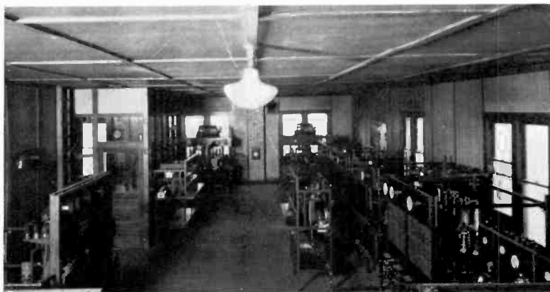
INFANT KDKA MATURES: INTERIOR OF PIONEER WESTINGHOUSE STATION
