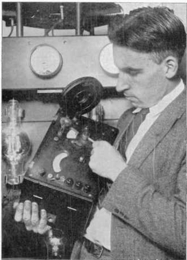
ADJUSTING WAVE LENGTHS WITH A WAVE METER AT W J Z, THE WESTINGHOUSE STATION AT NEWARK, NEW JERSEY
