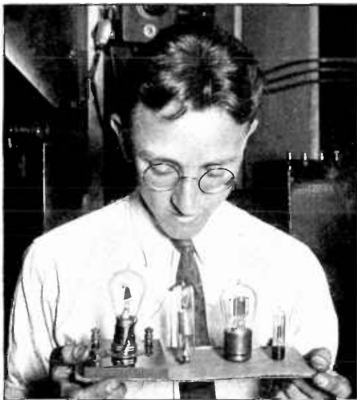
A CRYSTAL RADIO-RECEIVER IN THE FORM OF A NECKTIE-PIN INVENTED BY MR. C. SAUNDERS (RIGHT), AND A GROUP OF VACUUM TUBES FROM FLEMING VALVE TO PEANUT AUDION OR TRIODE.
