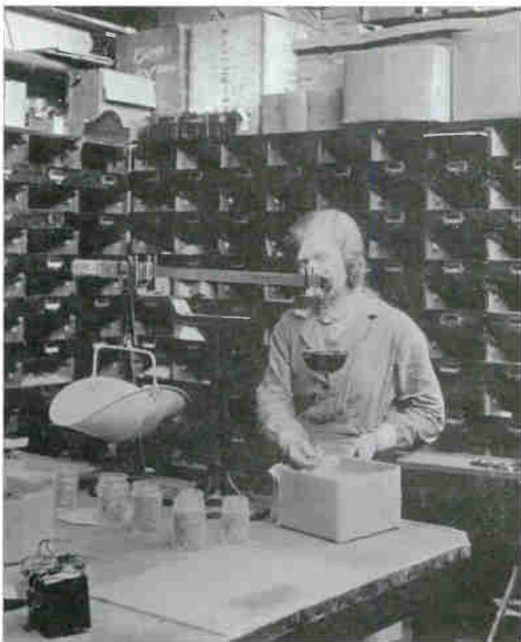
Pye Radio factory, 1932 Counting screws by weight
