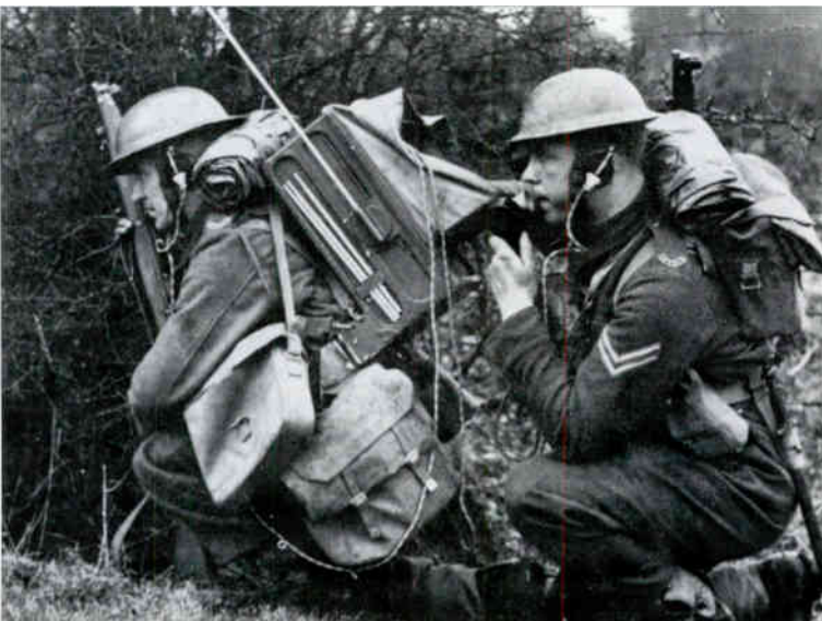
WS18 infantry pack set designed and manufactured by Pye
