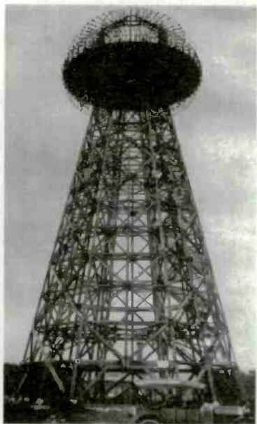
Tesla's Wardencllyffe Tower, completed in 1903, was intended for Radio broadcasting and wireless transmission of power across the Atlantic.
