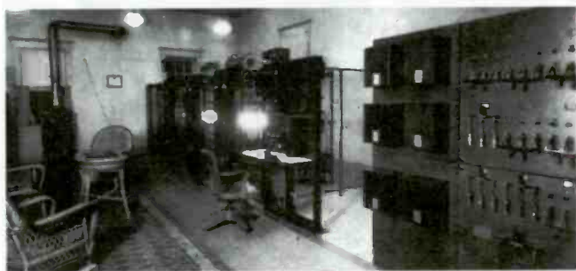
Early transmitter equipment at WFBM, circa 1927.
