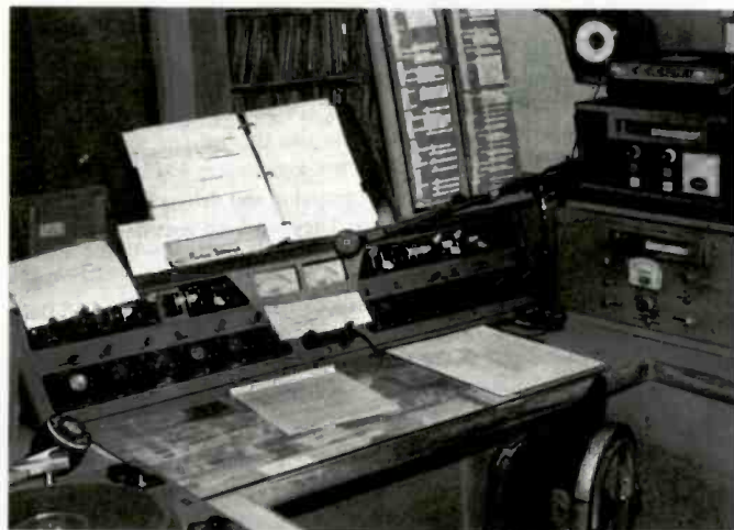
Typical control room for combo operator includes Gates Dualux Console, 1960s.
