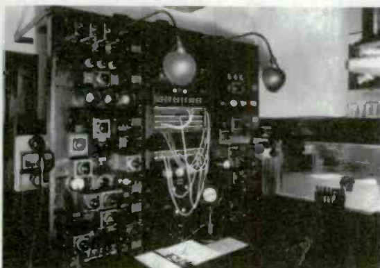
WBT Charlotte control room, circa 1929.
