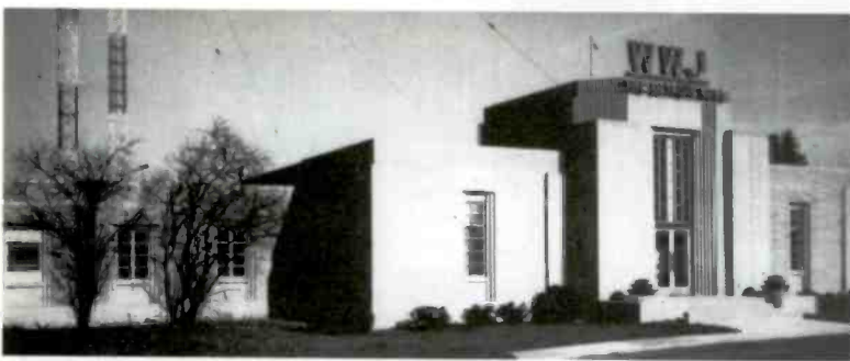
WWJ Detroit transmitter building, 1936.
