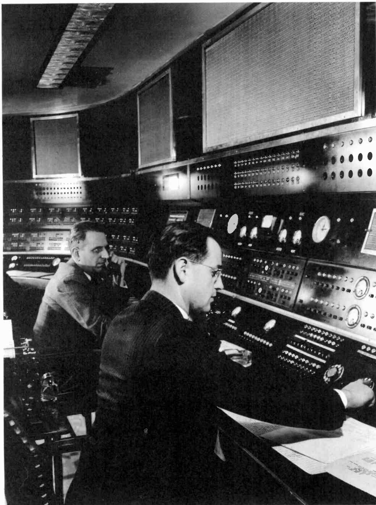
Master control desk. Part of the intricate equipment by which broadcasts are switched over a network.
