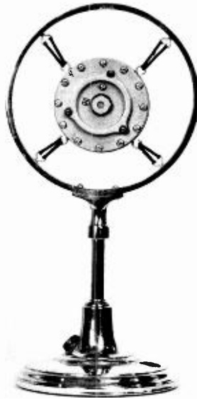
LATER FORM OF CARBON MICROPHONE
