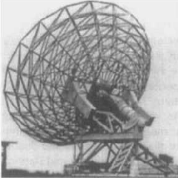
Figure 15.35. Beam waveguide feed system of the dual-reflector antenna of a ground-based satellite communication station (reproduced from [151], Circa 1961).
