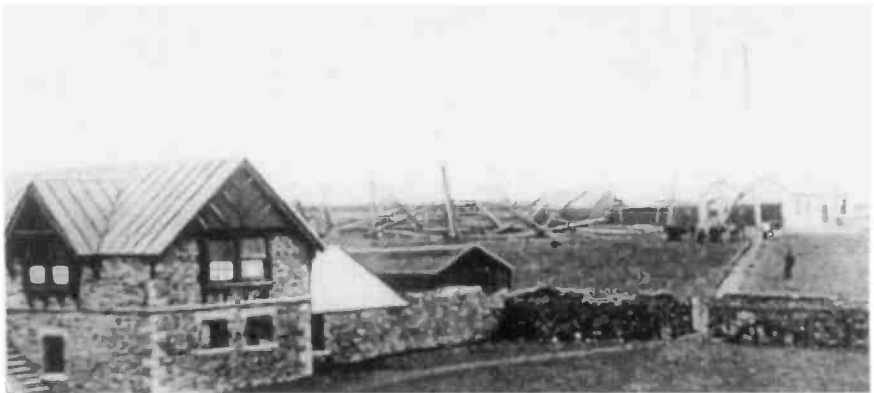
Figure 12.22b. Poldhu aerial systems: the effect of bad weather on the first aerial.
