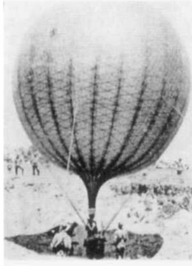
Figure 13.14 (left) A very early photograph illustrating the use of wireless telegraphy in wartime. These aerials hanging from balloons served radio transmitters and receivers operated by the Royal Engineers in South Africa.
