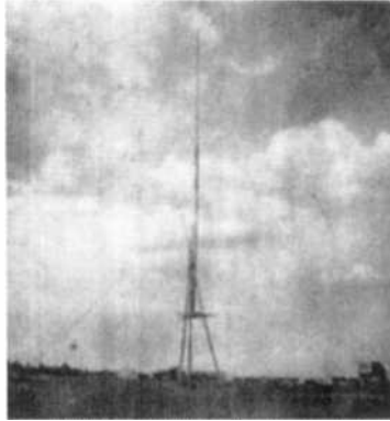
Figure 13.12. Early photograph of wireless telegraphy antenna believed to be at the Modder River encampment. This appears to have been constructed of bamboo poles, which caused problems because of splitting of the poles. (Photo reproduced by courtesy of the Royal Naval Museum, Admiralty Library Collection, MSS 277 Papers of Charles Beadnell).
