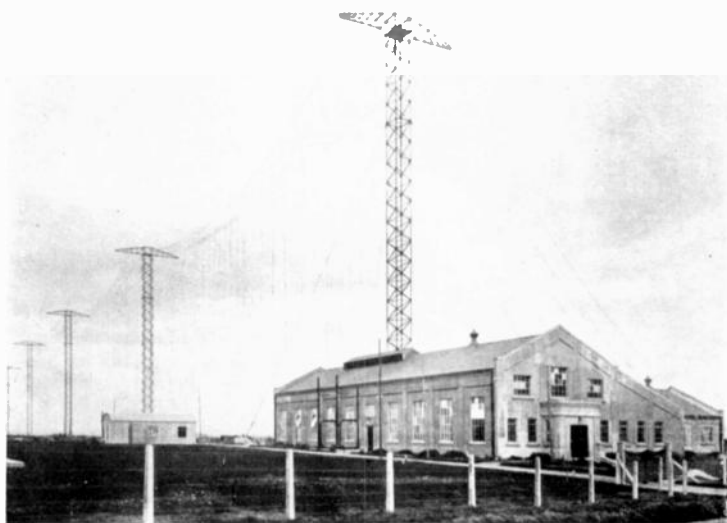
The Marconi Co.'s Beam Station, Dorchester. Power house building and offices, with 270-ft.-high masts.
