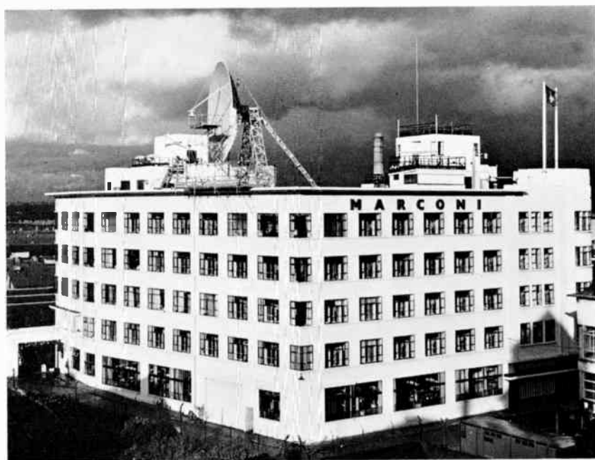
23. Part of Marconi House, Chelmsford, with thin-line tropo-scatter antenna on the roof
