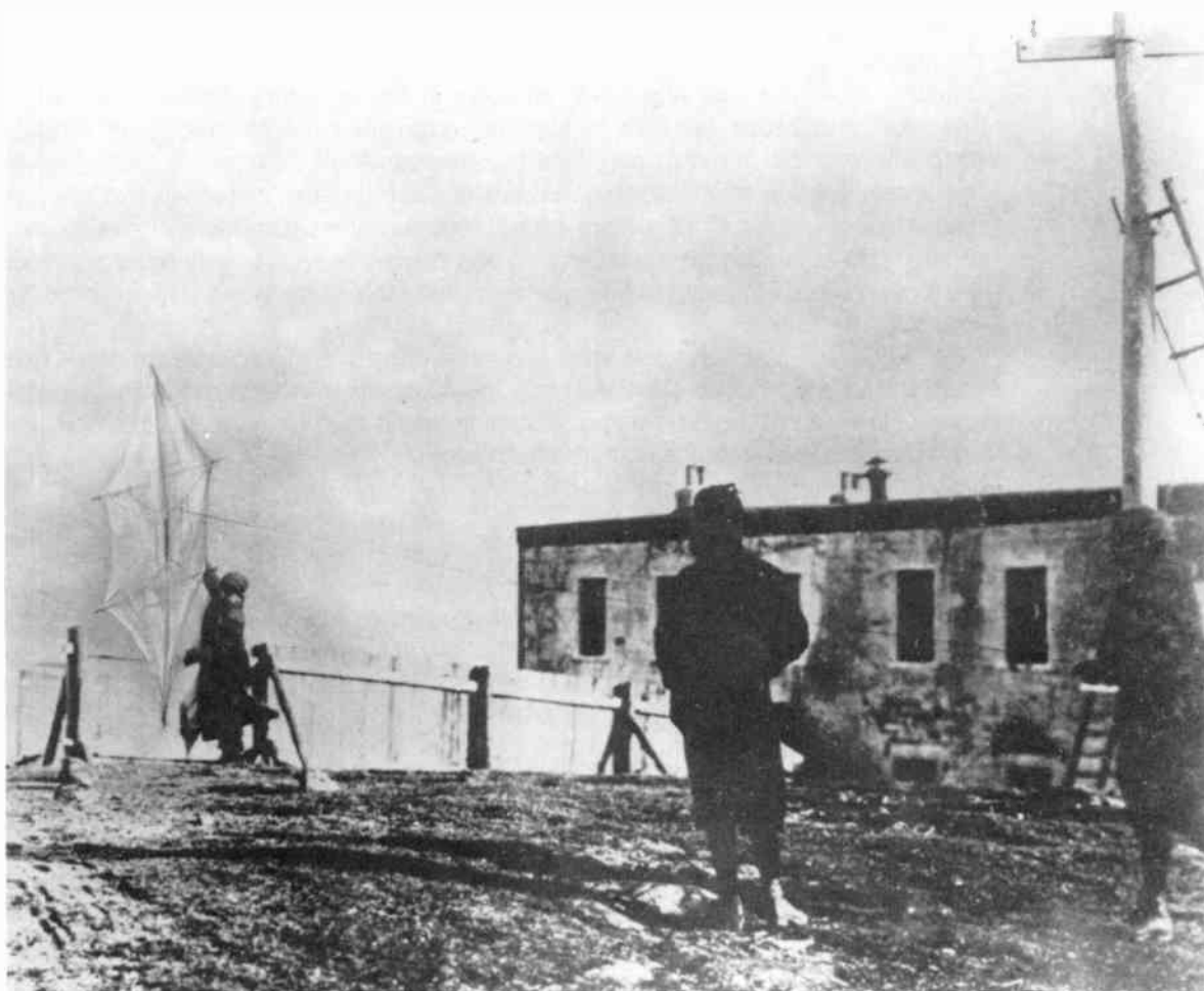
FIGURE 4-5. Marconi's Associates Launch an Antenna Kite at Poldhu
