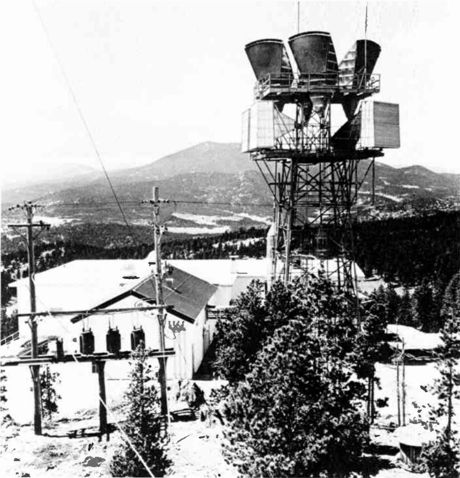
This microwave tower can send pictures, computer data, and telephone calls through the air in a very specific direction. This made possible coast-to-coast network television. (Western Electric.)
