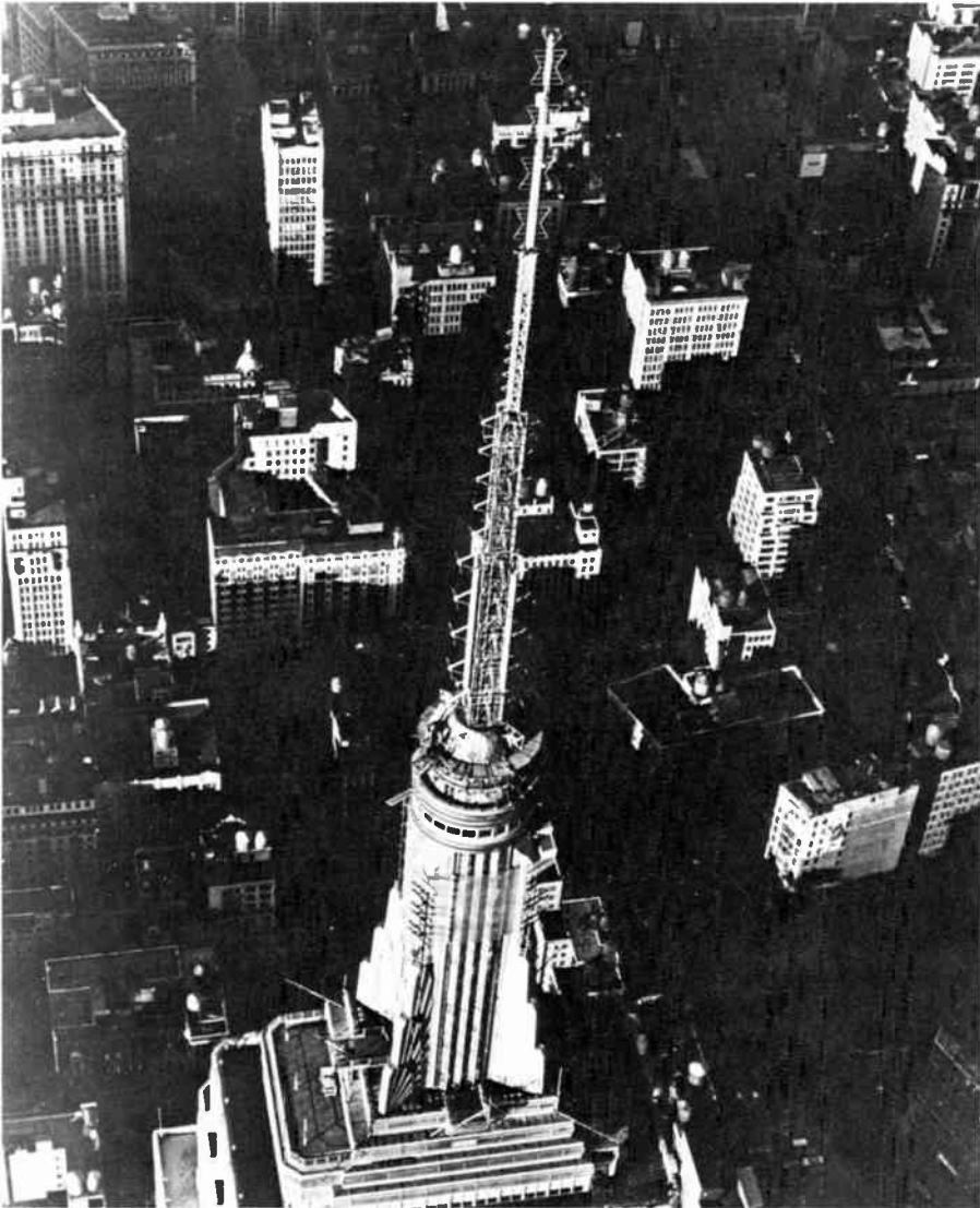
An antenna used by television stations in New York City to send television pictures through the air. This antenna is located on the Empire State Building. (Courtesy Empire State Building.)
