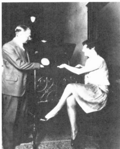
1929. Now working for RCA, Vladimir Zworykin demonstrates the kinescope, a cathode-ray TV receiver, which along with the iconoscope completes an all-electronic TV system.
