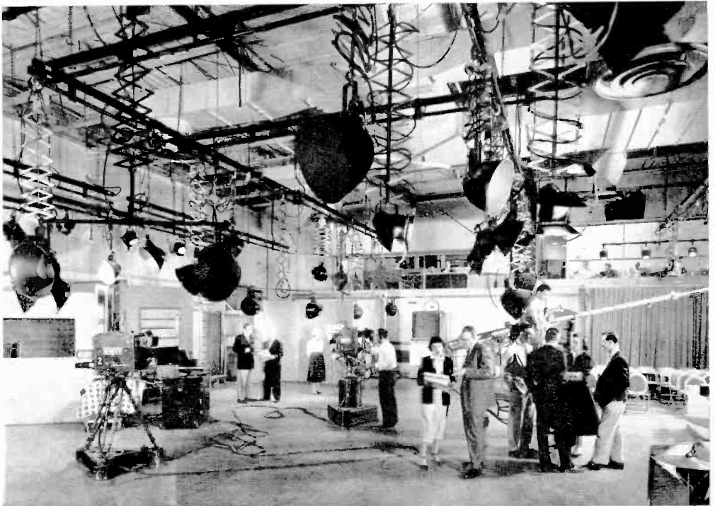
WHIO-TV Studio 2 is 50 feet wide by 63 feet deep. Control room is elevated.
