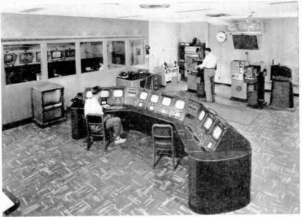
Design and construction of WHIO building and studios by The Austin Company
