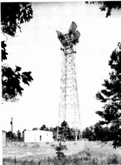
Fig. 3-5. A microwave relay station. Both coaxial cables and microwave relay facilities are provided by the Long Lines Department of the American Telephone & Telegraph Company for television and radio network service. Practically all routes are equipped for transmitting color. (American Telephone & Telegraph Company.)
