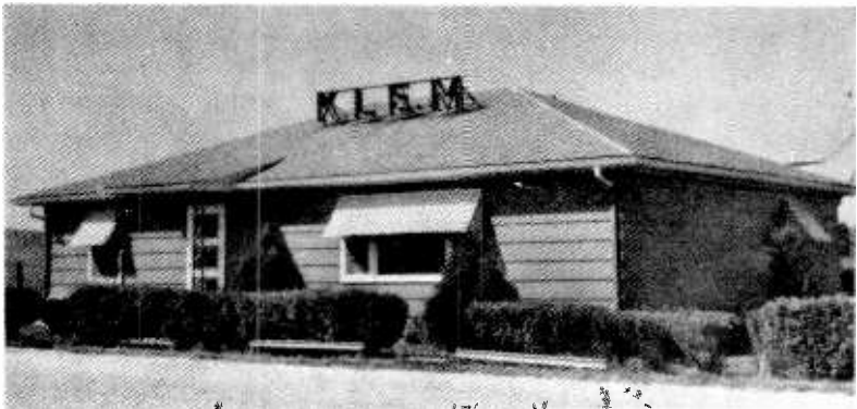
Fig. 6-10. A combined operation housed in what could pass for a residential building. This one was built in 1954 by a local contractor who planned to convert it to a residential property when the station failed! (1968 Photo courtesy of KLEM)
