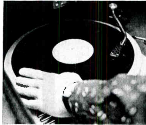
For a slip-cue start, the operator holds the record on a spinning turntable.
