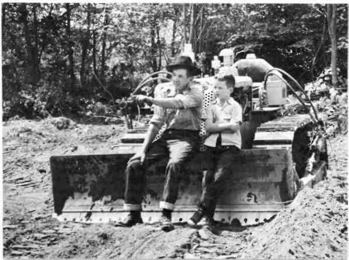
Murrow and Casey, with bulldozer, at Pawling
