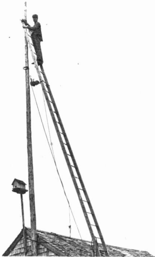
6. Harold Beverage erecting mast for his antenna on the pig sty building, Beverage farm, North Haven, Maine.
