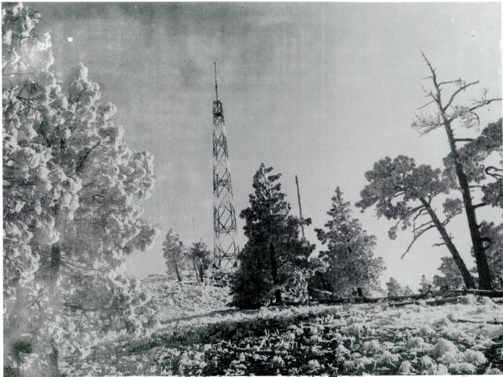
At Last! -- The Transmitting Tower is Raised
