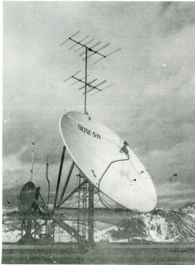
Some of CFJC's programming comes from satellites and there are two large receiving dishes located on the roof of Broadcast Centre.
