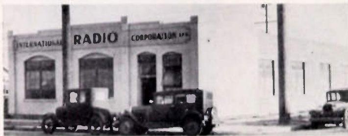
Factory of International Radio Company, manufacturers of the new "Westernaire" line.
