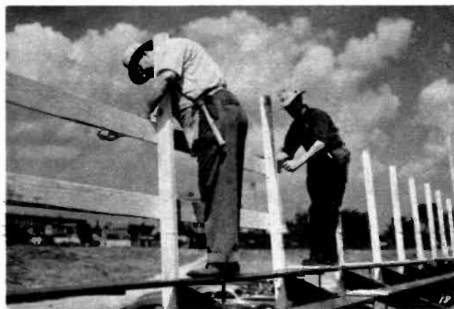
HUNDREDS OF HOURS MAY BE SPENT ON CONSTRUCTION ALONE
