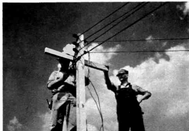
TELEPHONE MEN INSTALL LINES FOR THE PUBLIC ADDRESS SYSTEM
