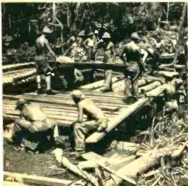
ENGINEERS CORPS: CONSTRUCTING A SAFE BRIDGE
