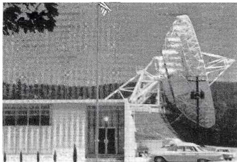
For hardware merchants, building ground stations such as this Hughes experimental system in Arkansas, will be where the big money is.
