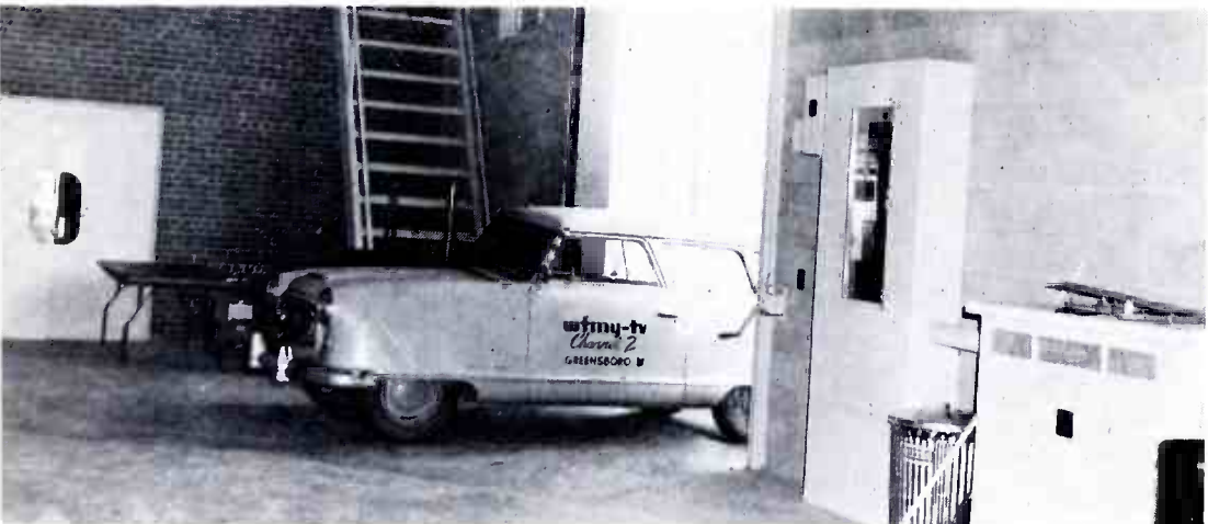
Delivery trucks can drive right into storage area, which totals 14,000 sq. ft. Need for such space sparked management's decision to build.
