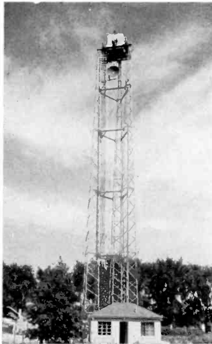
Relay equipment towers at Michigan City, Ind. A 6 foot parabolic reflector is seen being hoisted to its location on west wall of penthouse.
