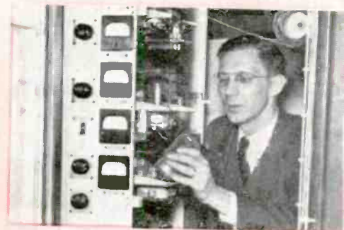
WALL-MOUNTED UNITS afford easy access to all tubes and wiring. Rear doors further increase ease of reaching all components. Illustration above shows portion of the aural transmitter's r-f driver unit.
