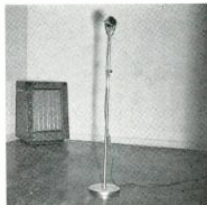
Echo chamber in the WIS studios, a 12-foot room with hard plaster on all walls and ceiling. Only units in the room are the speaker and microphones.
