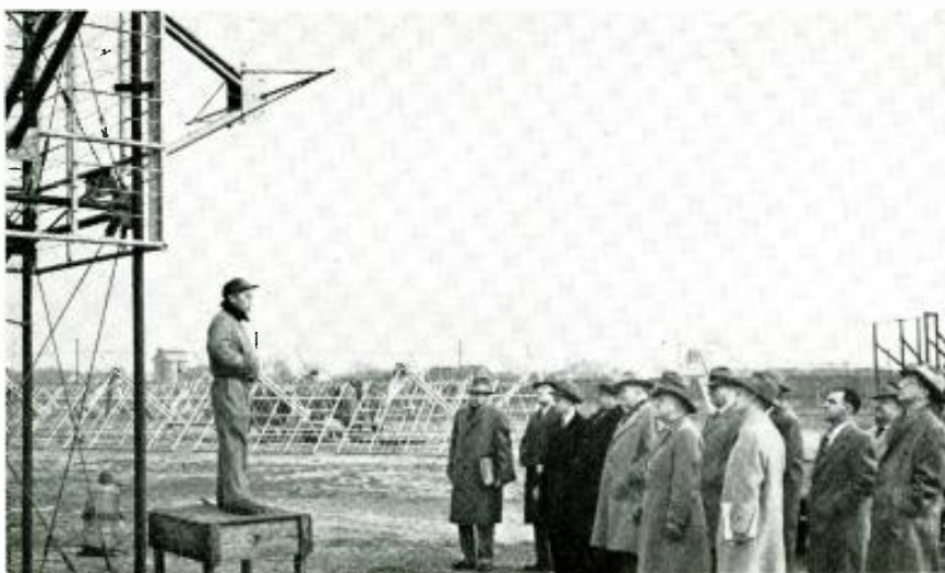
Howard E. King, RCA antenna engineer, reviewing a progress report on the 7-station FM/TV Empire State Building antenna, which is expected to be in full operation by early March, before a group of consultants who participated in a symposium dealing with practical considerations in the use of TV super-turnstile and super-gain antennas. The design and installation of the antenna will be analyzed in a nine-paper panel on Broadcast Day (March 20) at the IRE national convention at Grand Central Palace.
