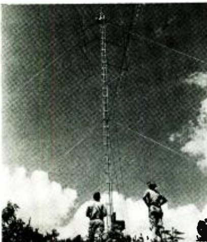
Below: Sixty-five-foot tower with three yags, cut for channels 4, 5 and 7, on mountain peak 1000' above Hazard, Ky. Installed to pick up programs from Huntington, West Virginia and Cincinnati, Ohio, 90 and 150 airline miles away. Right, below: View of poles on which have been mounted about 3000' of open-wire lead-in, feeding signals to amplifiers. At bottom of hill amplified signals are fed to coax cable mounted on poles of the local electric light company. From these poles, smaller coax cable, strung into each home, feeds sets. Amplifiers have been placed along the system at intervals to compensate for line losses in signal strength. Junction boxes, which can be mounted on any pole, permit four homes to be connected into the system from a single pole. At present, about 600 feet of the heavy cable has been strung on power company poles, and about twenty receivers have been installed. (Courtesy G.E.)
