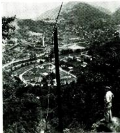
Below: Sixty-five-foot tower with three yags, cut for channels 4, 5 and 7, on mountain peak 1000' above Hazard, Ky. Installed to pick up programs from Huntington, West Virginia and Cincinnati, Ohio, 90 and 150 airline miles away. Right, below: View of poles on which have been mounted about 3000' of open-wire lead-in, feeding signals to amplifiers. At bottom of hill amplified signals are fed to coax cable mounted on poles of the local electric light company. From these poles, smaller coax cable, strung into each home, feeds sets. Amplifiers have been placed along the system at intervals to compensate for line losses in signal strength. Junction boxes, which can be mounted on any pole, permit four homes to be connected into the system from a single pole. At present, about 600 feet of the heavy cable has been strung on power company poles, and about twenty receivers have been installed. (Courtesy G.E.)
