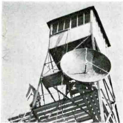
Figure 3 WMAL-TV pyramidal horn antenna as mounted on 7000-mc microwave relay transmitter.
