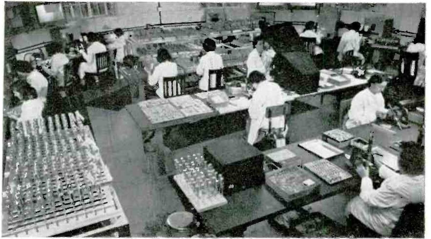
Final assembly of gun mounts. Cleanliness, humidity and temperature control are closely watched at this stage of gun construction.
